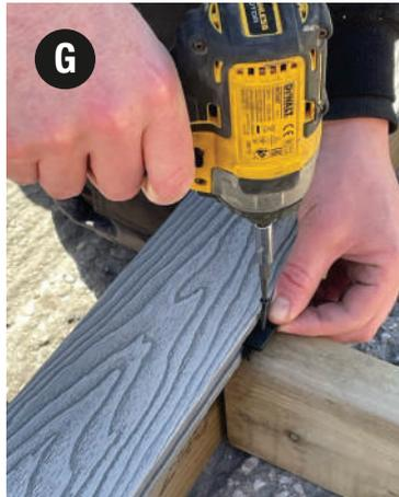
**H** Carry on laying your deck boards across the width of the deck using the plastic fixing clips.
