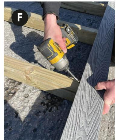
**G** Now screw the plastic fixing clips into the cross members (these clips space the boards perfectly).
