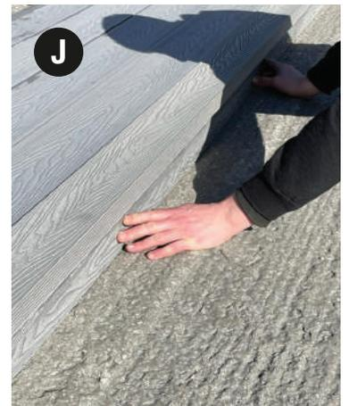
**K** There will be a slight gap between the deck boards and the nosings (this allows expansion)
